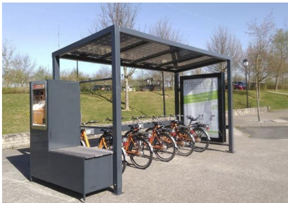
Picture 15. Covered parking lot with solar charging station for electric bicycles
